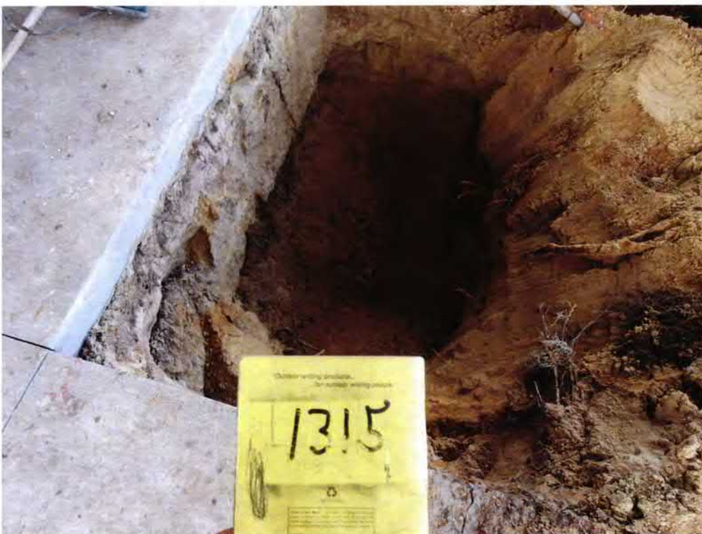
Picture 2: UST 1315Albatross excavation.
